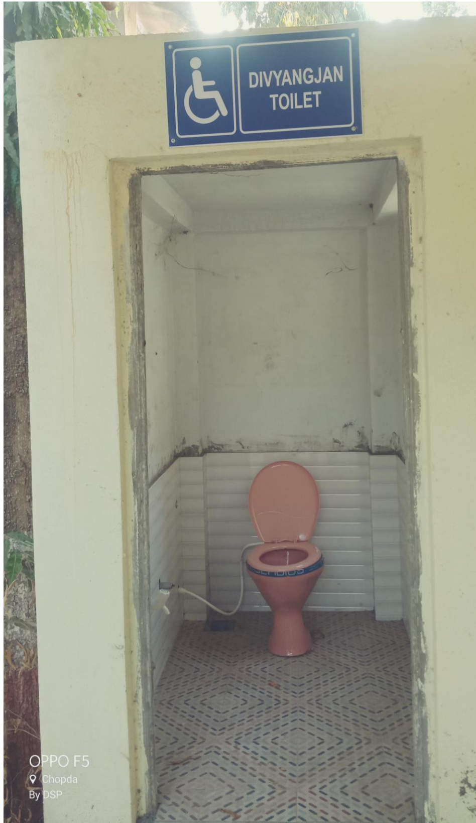
Divyangjan Friendly Toilet/ Washroom
